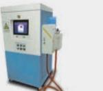
OPSE0Q4004  | Use the quick charger at public charging station                                 | Approx. 33 min (50 kW, room temperature) (Can be charged to 94%)                                               |
